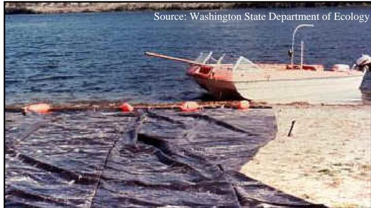
Bottom screening material being prepared prior to installation around a boat dock
