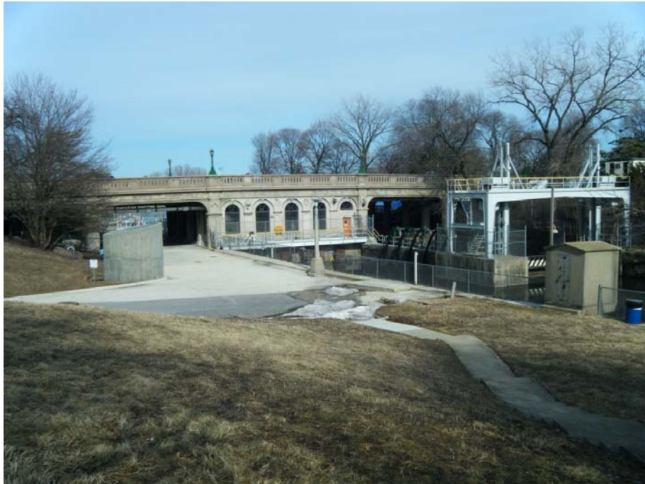
Figure 8. Wilmette Pumping Station
