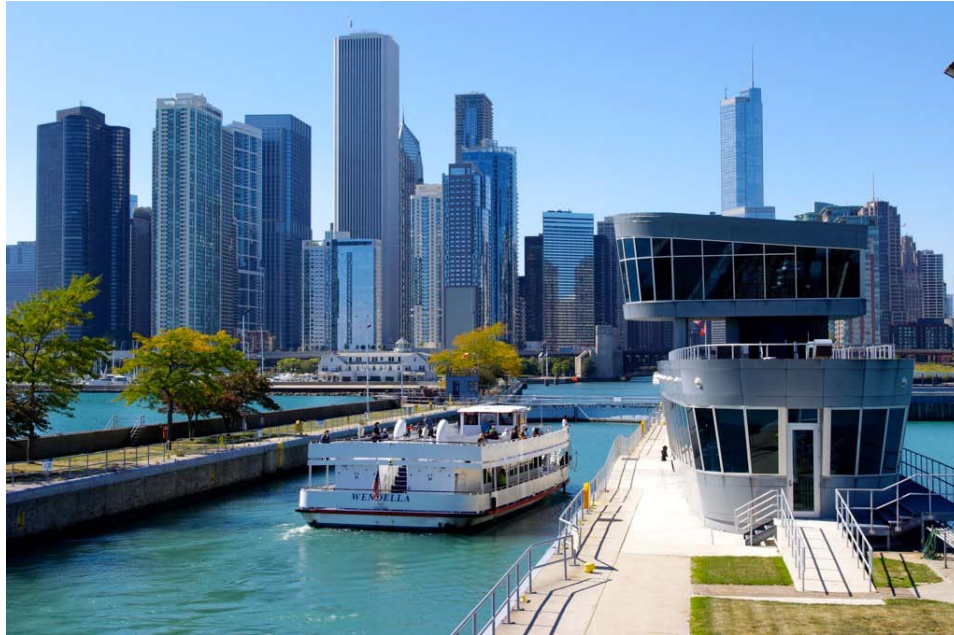
Figure 4. Chicago River Controlling Works Lock
