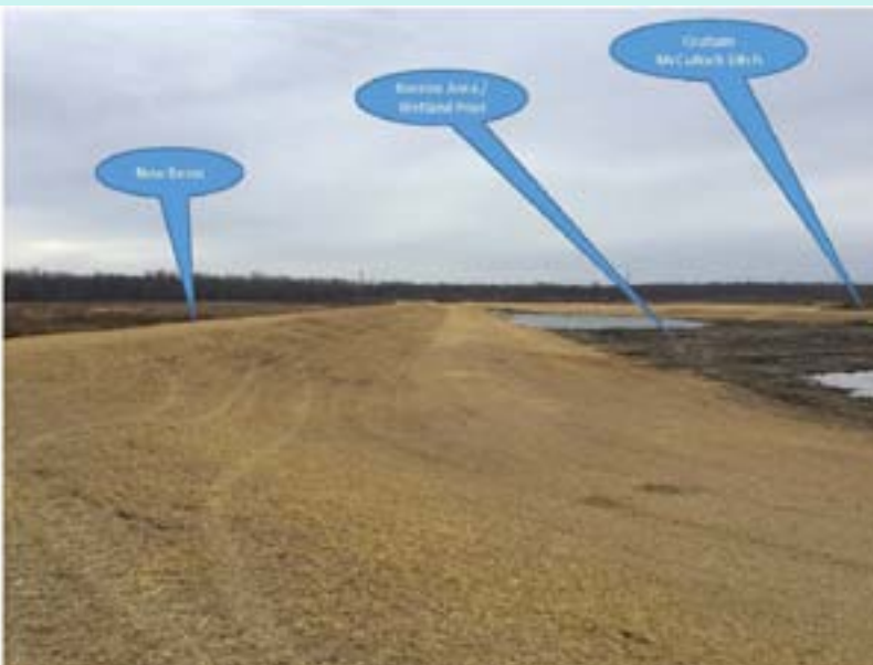
The Eagle Marsh project created an earthen berm across the floodway to prevent mixing of the watersheds at the 100-year flood level. The first phase was completed in fall 2015.
