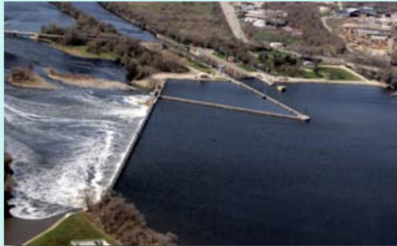
Aerial view of Brandon Road Lock and Dam, Joliet, Ill., April 22, 2014. The lock has been operational since 1933.
