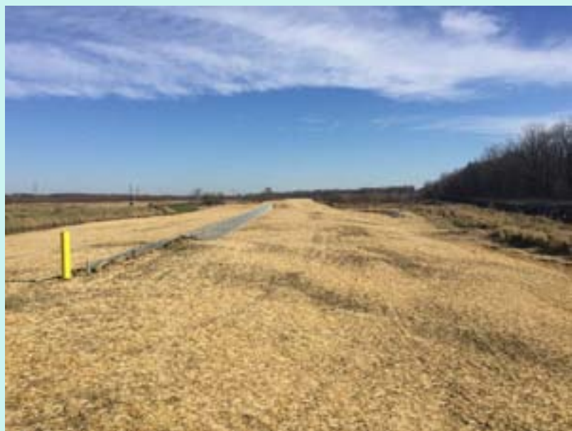
Notched berm with screening to stop Asian Carp transfer. The second phase, scheduled for 2016, will consist of removing the screen and filling the notch. This phase cannot be completed until all flood risk in the area has been mitigated.
