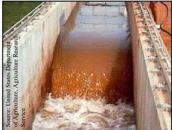
**Accelerated water velocity channels must be smooth to prevent the formation of low velocity flow zones near the walls.**
